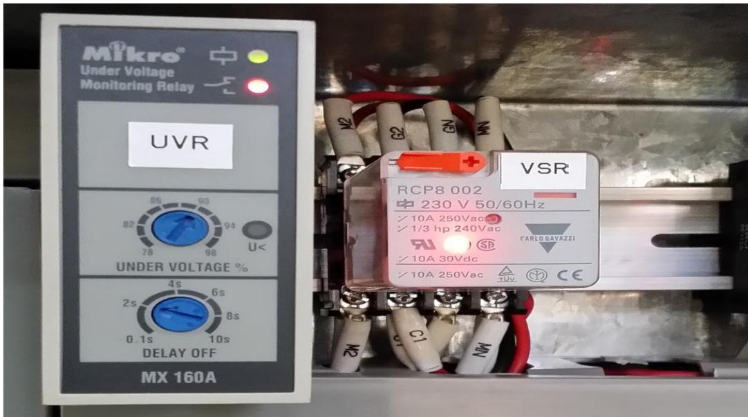
Figure 8.3 Changing the voltage threshold and time delay
