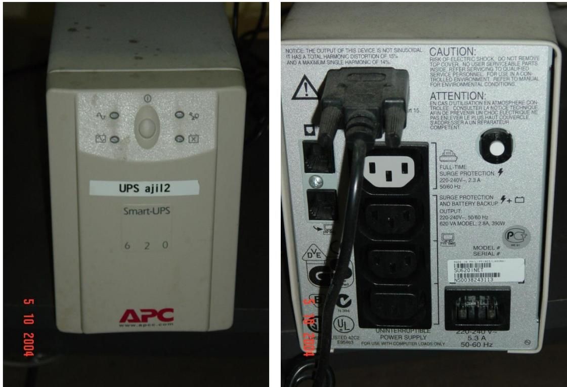
Figure 8.12 A Single Phase Uninterruptible Power Supply (UPS)
