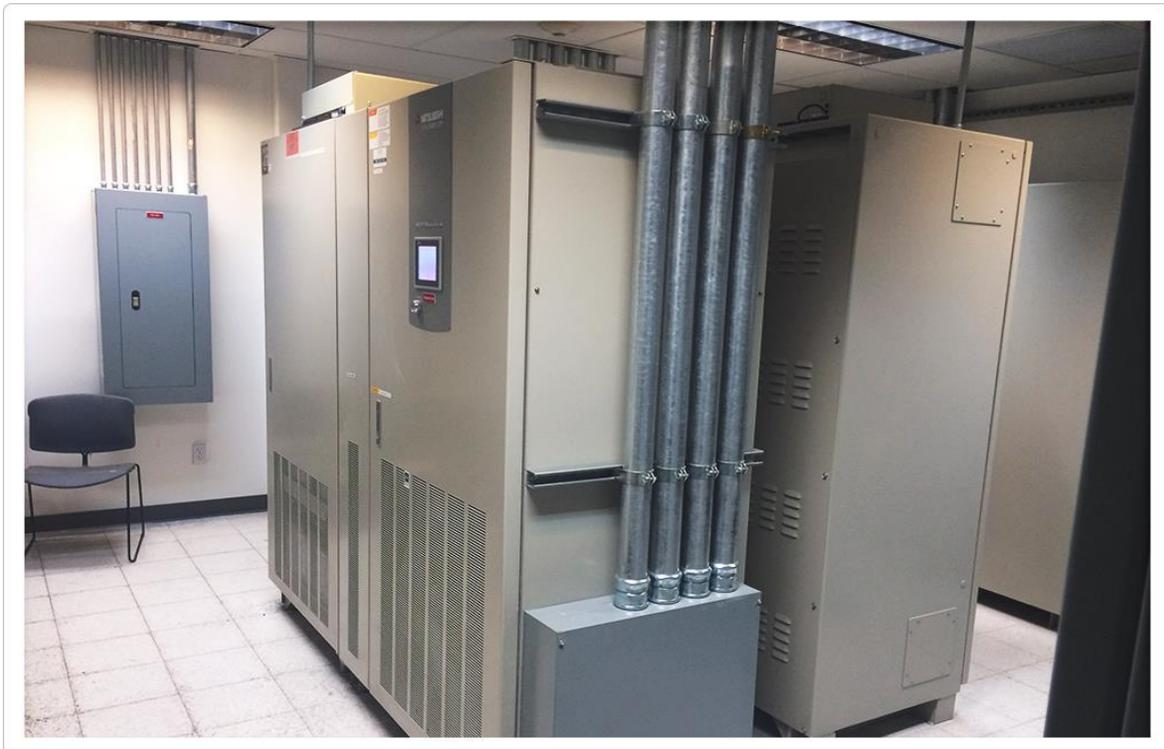
Figure 9.2 Three Phase Uninterruptible Power Supplies (UPS)
