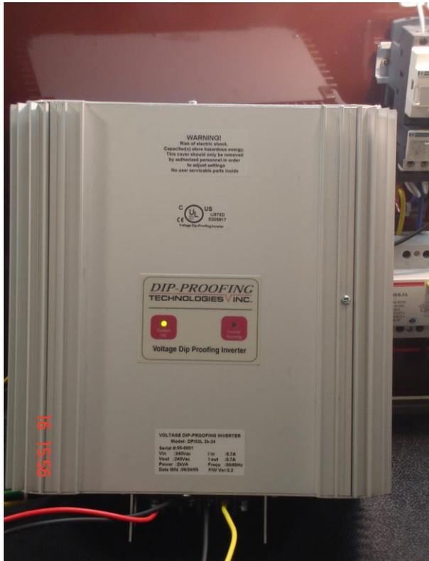
Figure 8.14 Dip Proofing Inverter (DPI)
