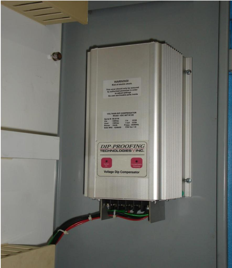
Figure 8.15 Voltage Dip Compensator (VDC)
