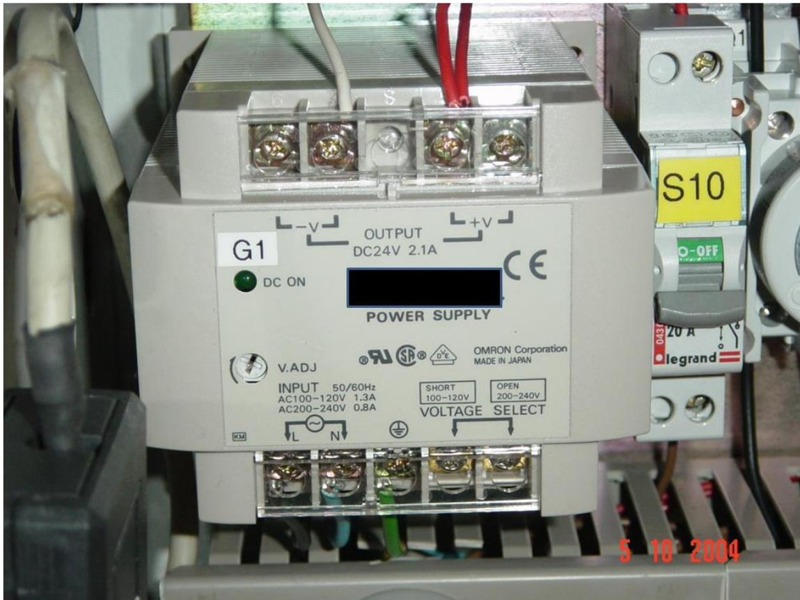
Figure 8.2 Example of a SEMI F47 compliance power supply
